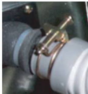
Figure 91: Flexible Drain Hose Connection.
